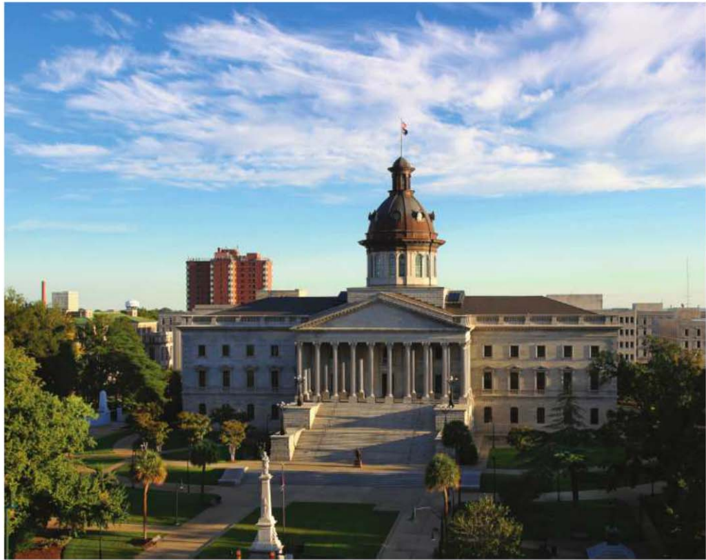
ABOVE: The copper-domed South Carolina State House.
